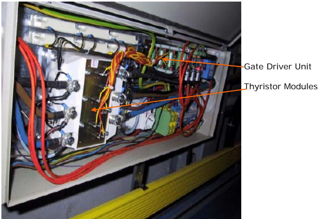
Depending on the installation one or two switches are included in one box.
